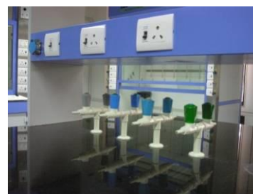
service valves & electrical sockets
